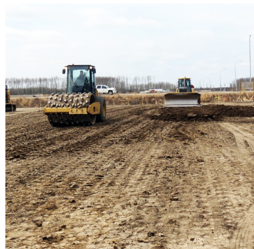
Infilling in progress.
