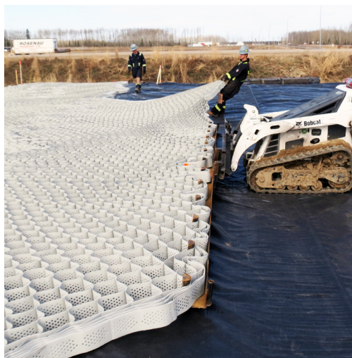
Installation of ToughCell® over geotextile.
