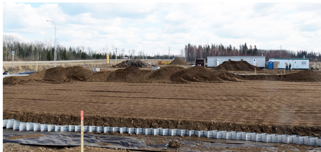
Yard area infilled and surfaced with gravel.
