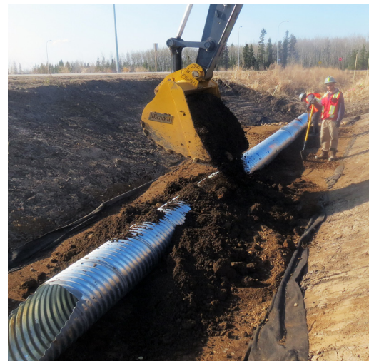
Preparation of drainage ditches.
