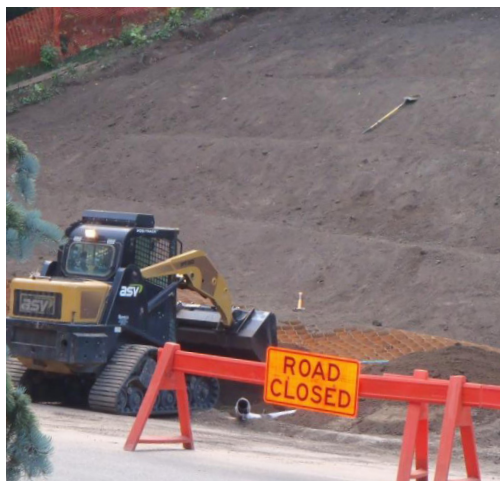
Infilling of Tough Cell® geocells
