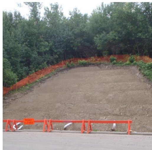
Graded and terraced slope
