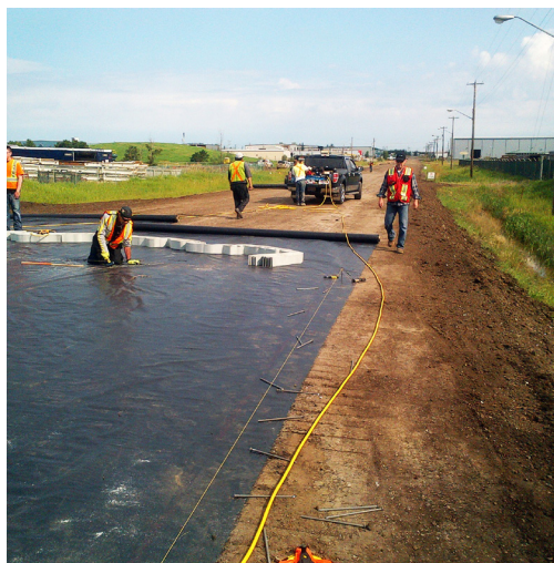
Woven geotextile installed as a separator between the base and subgrade
