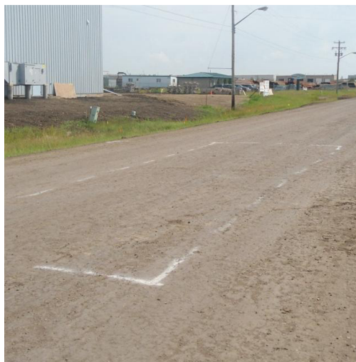
Pre-existing road marked with proof-rolled weak spot
