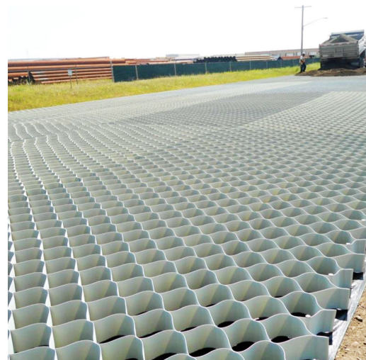
Installed Tough Cell® geocells
