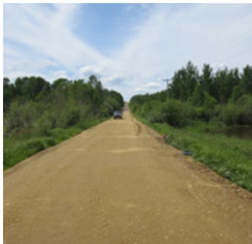
Completed road, June 2013
