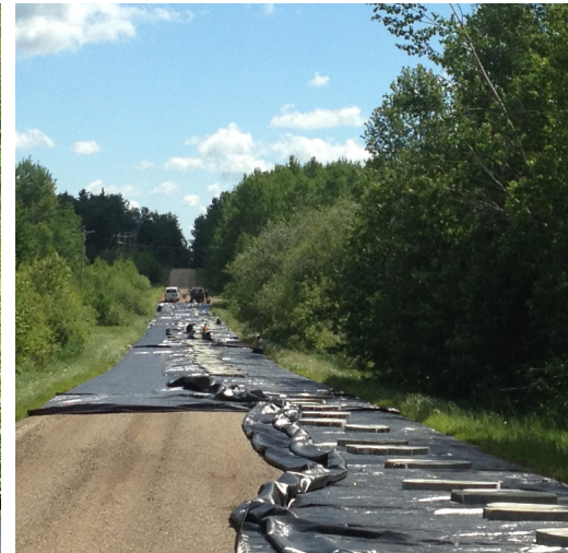
Installation of geotextile layer
