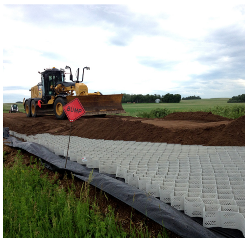
Infilling of Tough Cell® geocells
