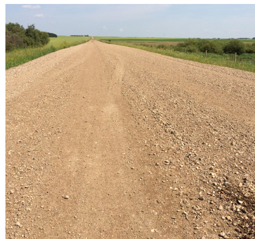
Completed road after rehabilitation
