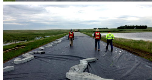
(top) Installation of geotextile to ground (bottom) Tough Cell® preparing to be stretched
