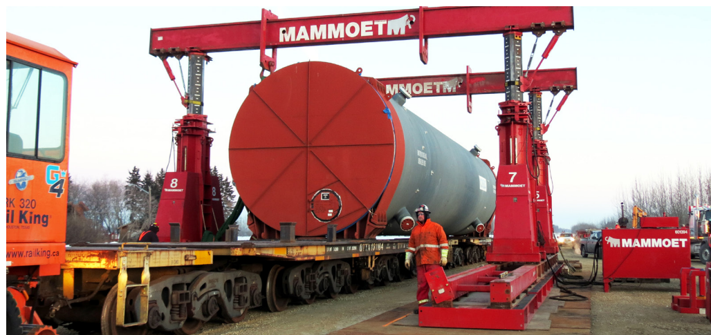
Crane installed and in operation.
