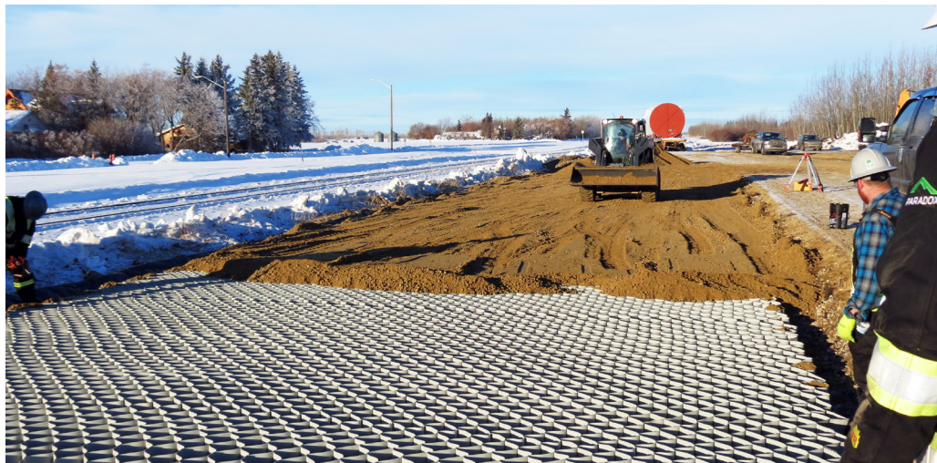
Installation and infilling of Tough Cell®
