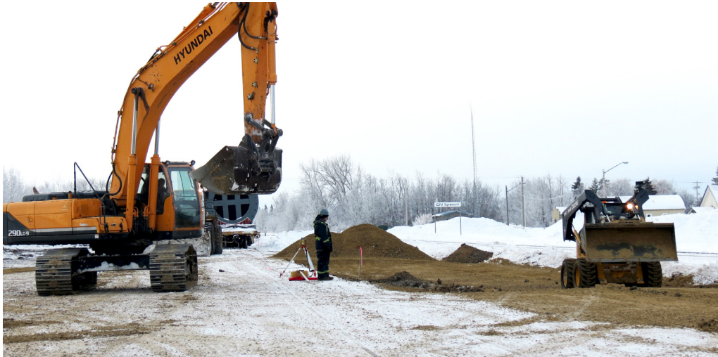
Preparation of base during winter conditions.
