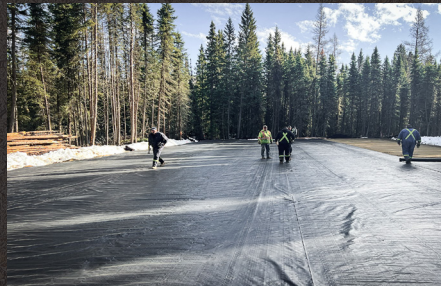
Laying geotextile.
