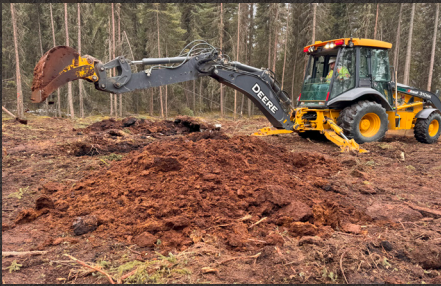
Site logging, clearing and preparation.
