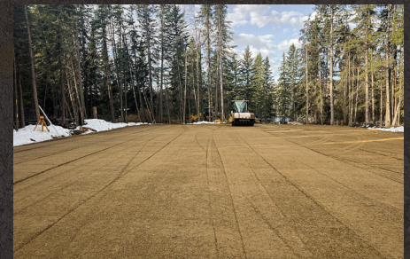
Compacting the top layer of Tough Cell®.
