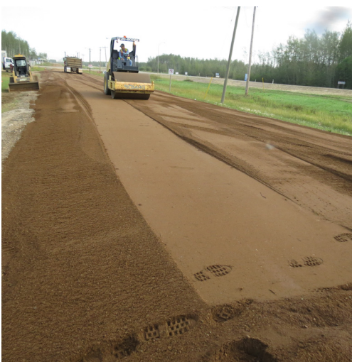
Compaction of sand base
