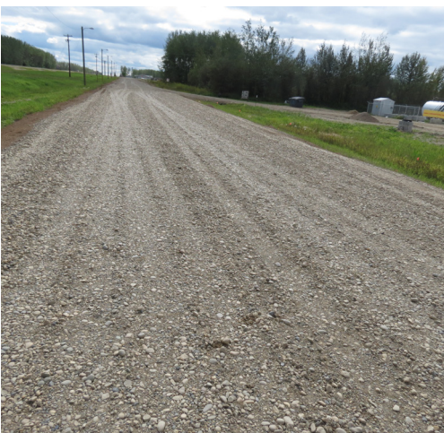
Completed road, August 2013
