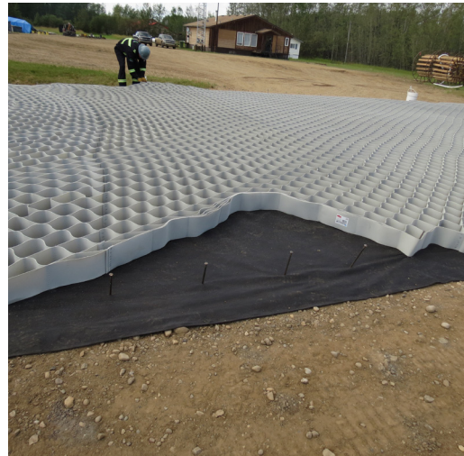
Installation of geotextile and Tough Cell®
