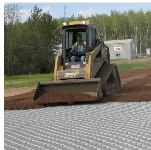
Infilling of ToughCell® with track loader
