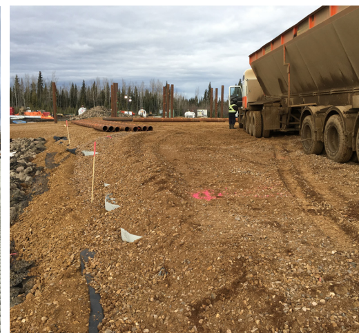
Gravel course and compaction
