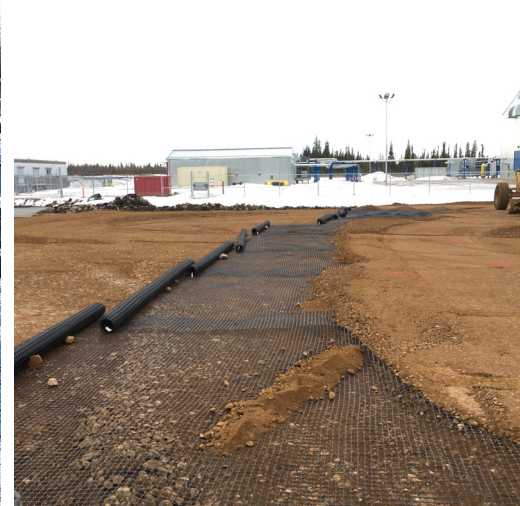
Installation, fill and compaction of geogrid layer
