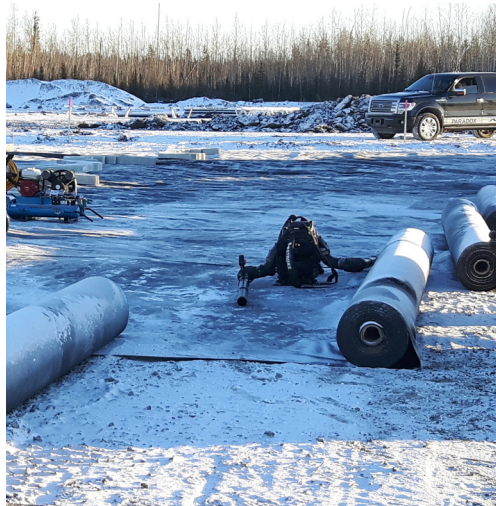
Installing geotextile in winter conditions
