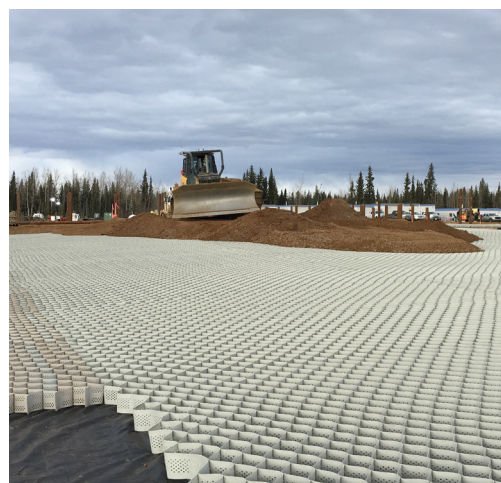
Infilling of Tough Cell® Geocells
